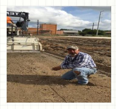
Vibratory compaction using Steel wheel
