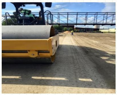
Grading to final lines and elevation
