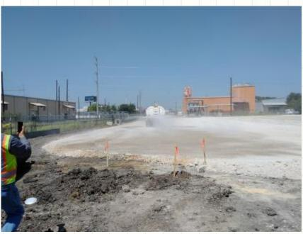
Reclaimer mixing together clay soil, CKD and Stabilizer
