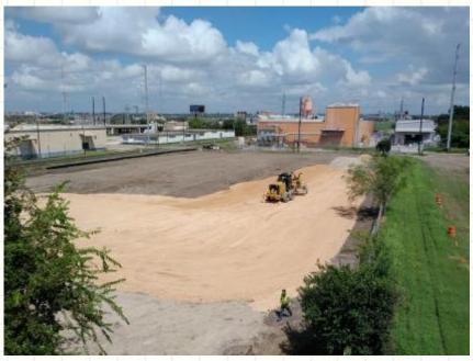
Cement Kiln Dust spread at 4% dry weight of soil
